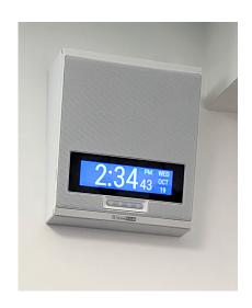
THE COMMUNICATION SYSTEM WAS DESIGNED WITH AN AtlasIED IP-SDM IPX SERIES LOUDSPEAKER AND AN LCD DISPLAY, INSTALLED IN EACH CLASSROOM.
