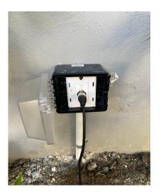
TO PROVIDE A SOLUTION FOR CASA DE CAMPO, ATMOSPHERE A-XLR REMOTE AUDIO INPUTS WERE INSTALLED AT TWO REMOTE LOCATIONS AROUND THE POOL INTENDED FOR THE MUSICAL TALENT.
